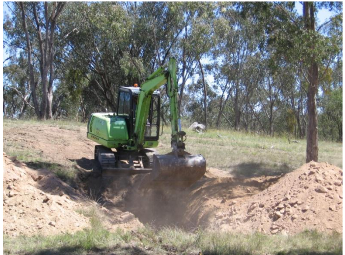
Figure 3: Infilling sampled pits using a small, 4.5t excavator prior to rehabilitation of the surface
