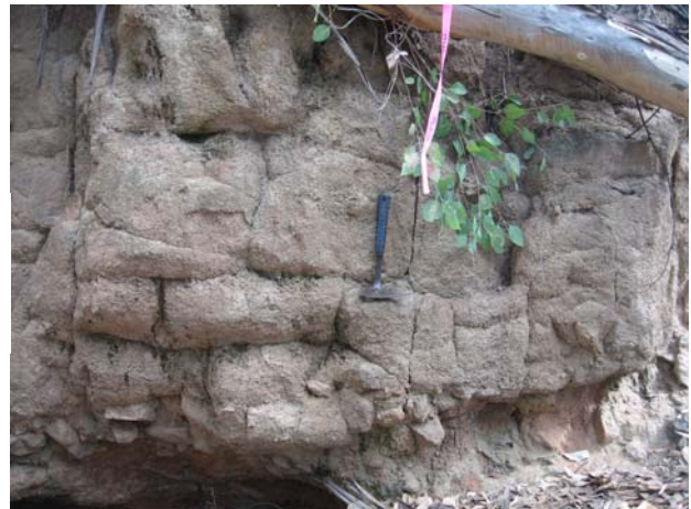
Figure 4: Exposed face in the Karaula Lead; a sample from the centre of this exposure assayed 0.5kg/cu m of tin
