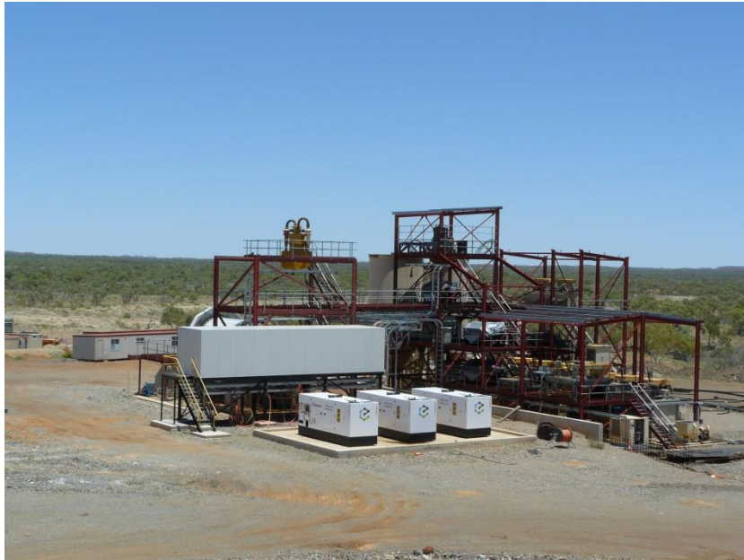
Lorena Concentrator Plant
